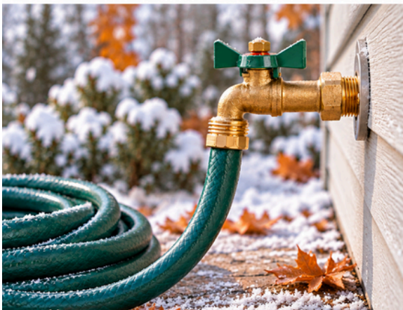
Hose attached · Bibb exposed
